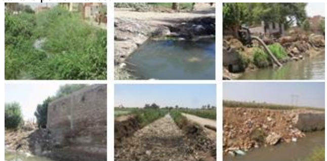
Photo 1: Bahr Awlad Mohamed Problems before rehabilitation
