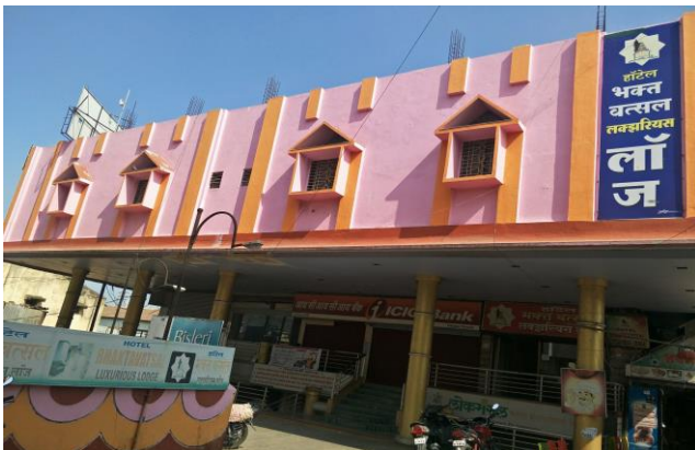
Fig.1 Front view windows with chajja and vertical fins (Site photograph)
