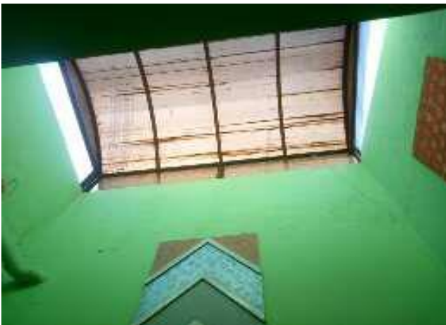
Fig.6 Air ducts view from inside (Site photograph)
