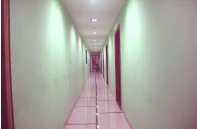
Fig.5 Passages connecting windows and air ducts. (Site photograph)
