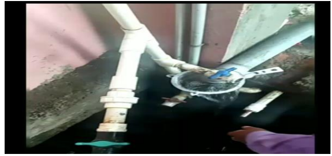
Fig.8 Rain water harvesting works (Site photograph)
