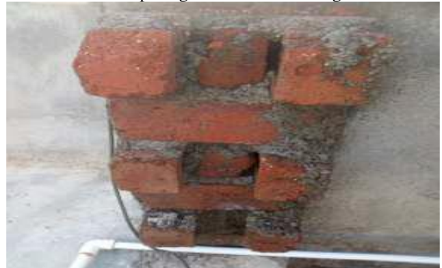
Fig.3 Rat trap bond (Site photograph)
