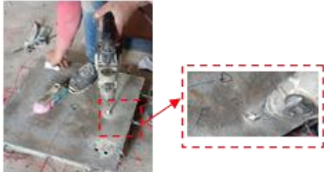
Fig. 5: Drilling method from the slab
